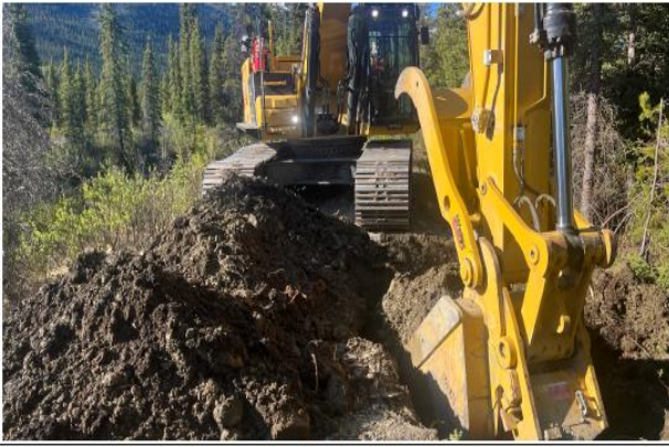
Picture 1: Crew digging a test pit
